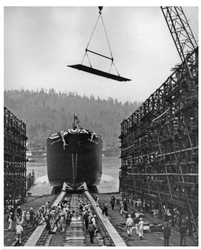
FIGURE 10 LAUNCH OF US CARGO SHIP, SS WILLIAM CLARK, USING RAILS IN 1942
