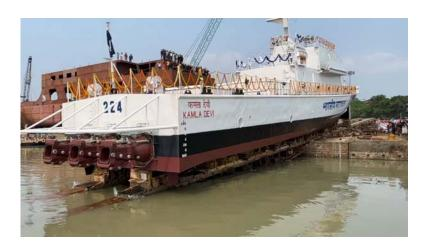
FIGURE 1 END LAUNCH OF FAST PATROL VESSEL, ICGS KAMALA DEVI, AT TITAGARH RAIL SYSTEMS LIMITED (KOLKATA) ON THE BANKS OF HOOGHLY RIVER. THE SLIPWAYS CAN BE SEEN BELOW THE SHIP.
