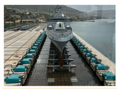
FIGURE 9 EXAMPLE OF A SYNCROLIFT
