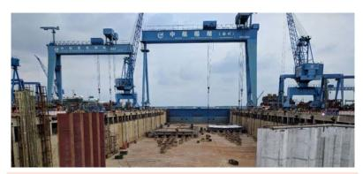
FIGURE 4 DRY DOCK AT AVIC DINGHENG SHIPBUILDING CO. LTD. , YANGZHOU, CHINA. TWO SHIPS UNDER THE ASSEMBLY PHASE CAN BE SEEN IN THE PICTURE WITH A DOCK GATE AT THE END.
